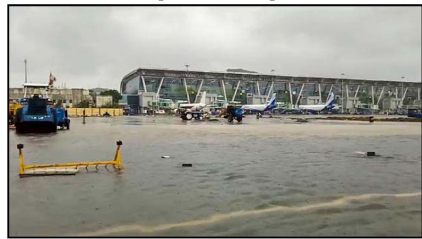
A rainwater drainage project, designed at a cost of Rs. 22 crore to prevent waterlogging on the Chennai Airport runway during the rainy season, has stalled due to a delay in the allocation of funds by the Airports Authority of India.
